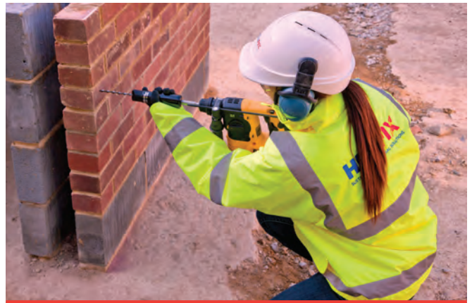
DryFix tie being power-driven into pilot hole
