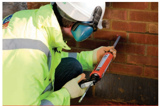
Injecting PolyPlus resin into near leaf to complete the ResiTie installation
