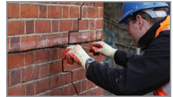
4. Using the HeliBar Insertion Tool push one HeliBar into the grout to obtain good coverage
