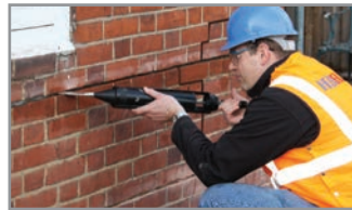
3. Using the Helifix Pointing Gun, inject a bead of HeliBond along the back of the slot
