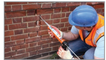
6. Inject CrackBond TE3 into the crack leaving enough space for making it good. Re-point the bed joints with matching mortar and make good the crack.
