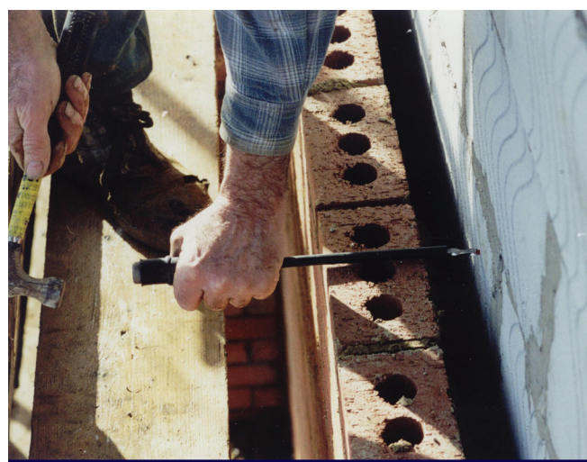
Installing TurboTie into aircrete blocks
