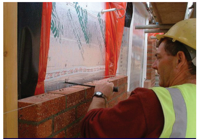
Installing TimTie through insulation into timber stud
