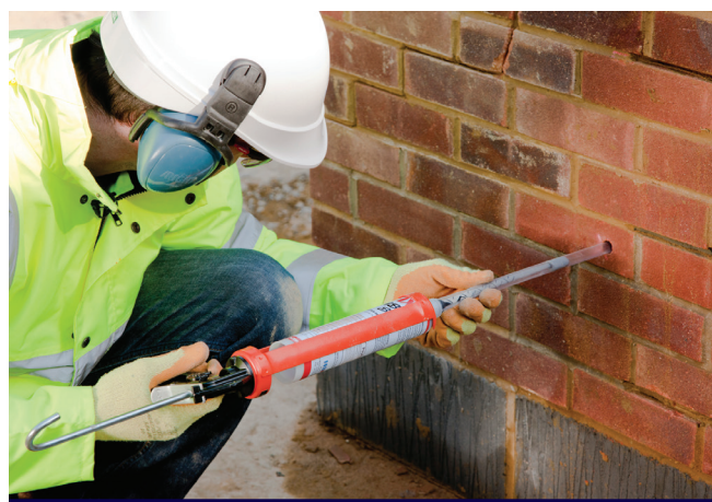
Injecting resin to complete the RetroTie installation
