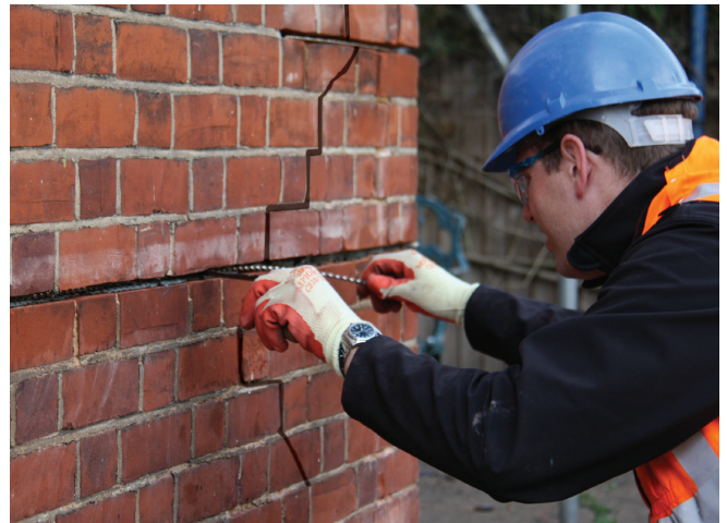
HeliBar is inserted into HeliBond grout within a cut slot. Used in pairs to form a masonry beam (Helibeam)
