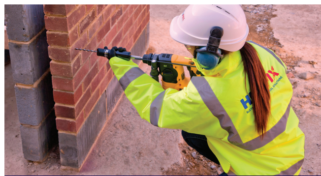
DryFix tie being power-driven into pilot hole
