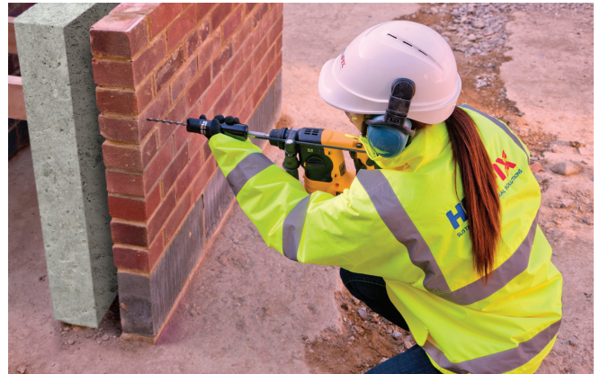
DryFix tie being power-driven into pilot hole
