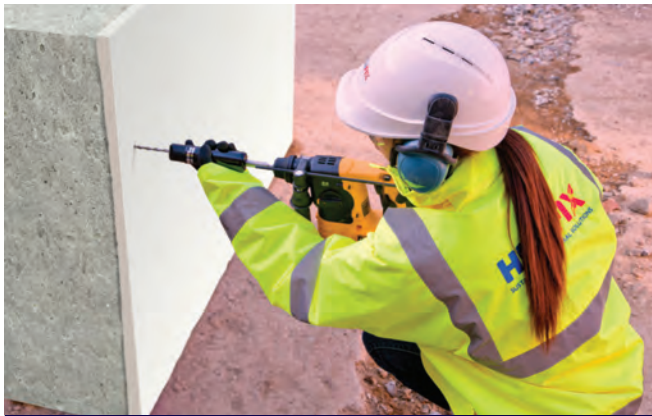
RenderPin being power-driven into pilot hole
