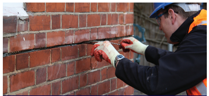
HeliBar is inserted into HeliBond grout with a cut slot
