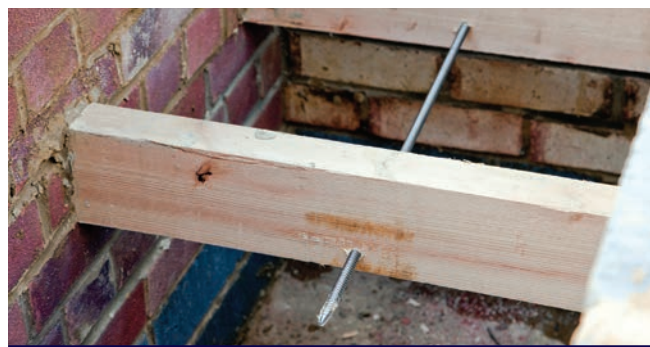
BowTie HDs installed through parallel floor joists
