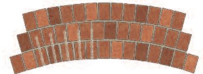
Masonry Arch Pinning of Debonded Bricks using DryFix
