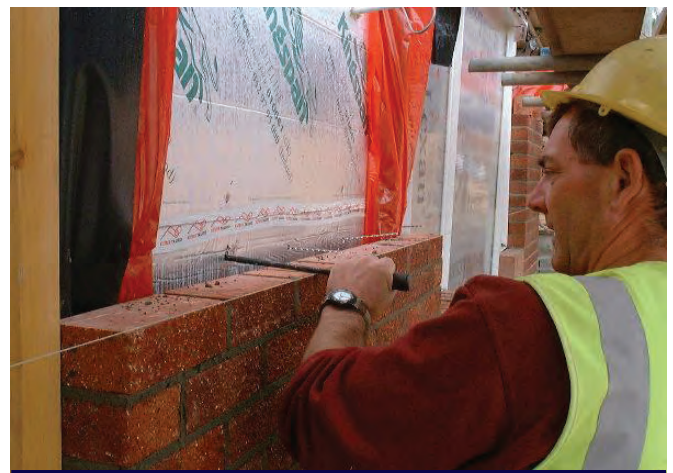
Installing TimTie through insulation into timber stud
