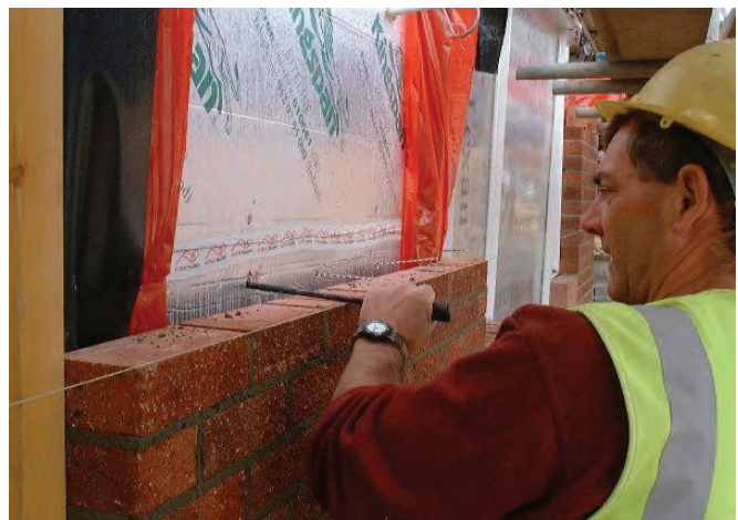
Installing TimTie through insulation into timber stud
