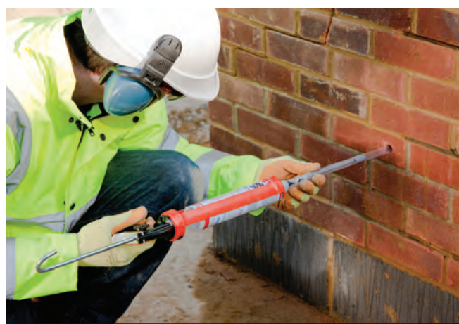
Injecting resin to complete the RetroTie installation
