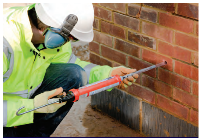
Injecting resin to complete the RetroTie installation
