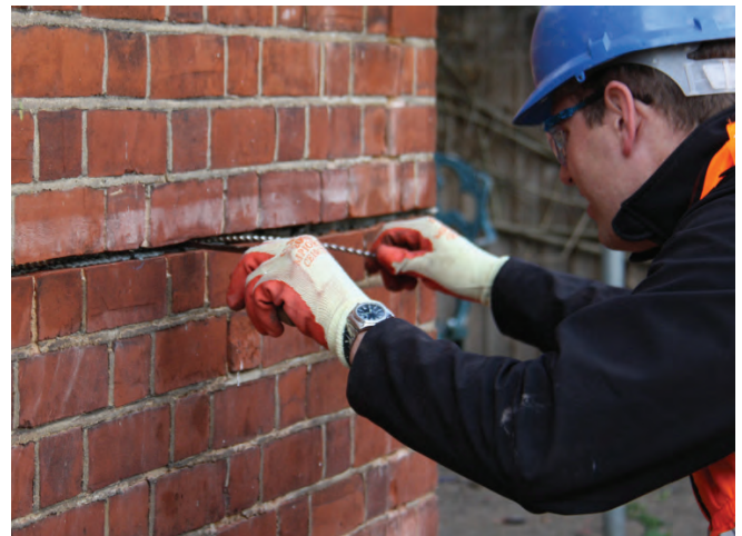
HeliBar is inserted into HeliBond grout within a cut slot. Used in pairs to form a masonry beam (Helibeam)
