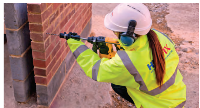
DryFix tie being power-driven into pilot hole
