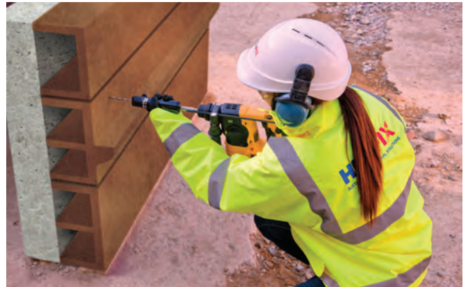
DryFix tie being power-driven into pilot hole
