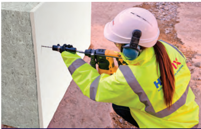
RenderPin being power-driven into pilot hole
