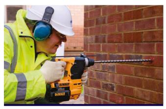
Drilling clearance hole in both leaves ready for CemenTie installation
