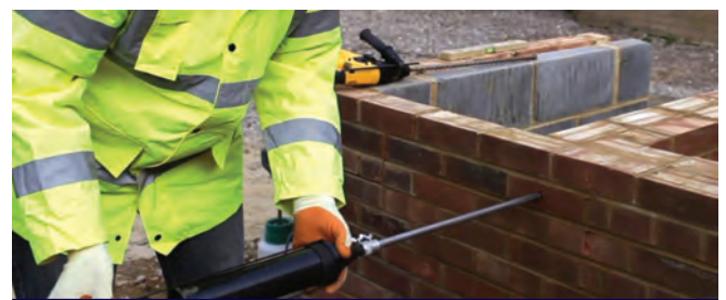
Inserting the grout-filled pinning nozzle, containing the CemTie, into the clearance hole
