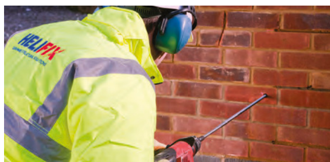
Drilling clearance hole for installing BowTie into joist end
