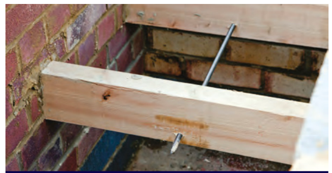
BowTie HDs installed through parallel floor joists
